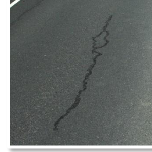
Reflection Crack
