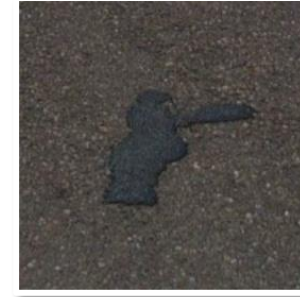
Bitumen Repair
